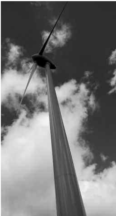
Above: A wind tower
