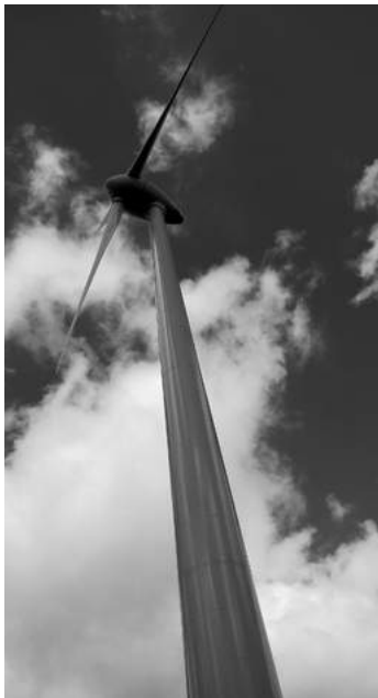
Above: A wind tower
