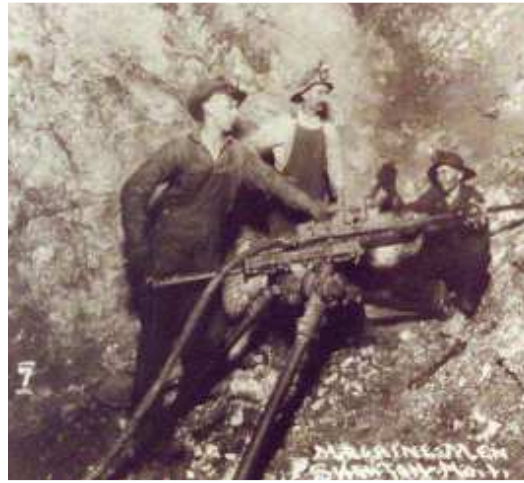
Man using a jackleg drill
