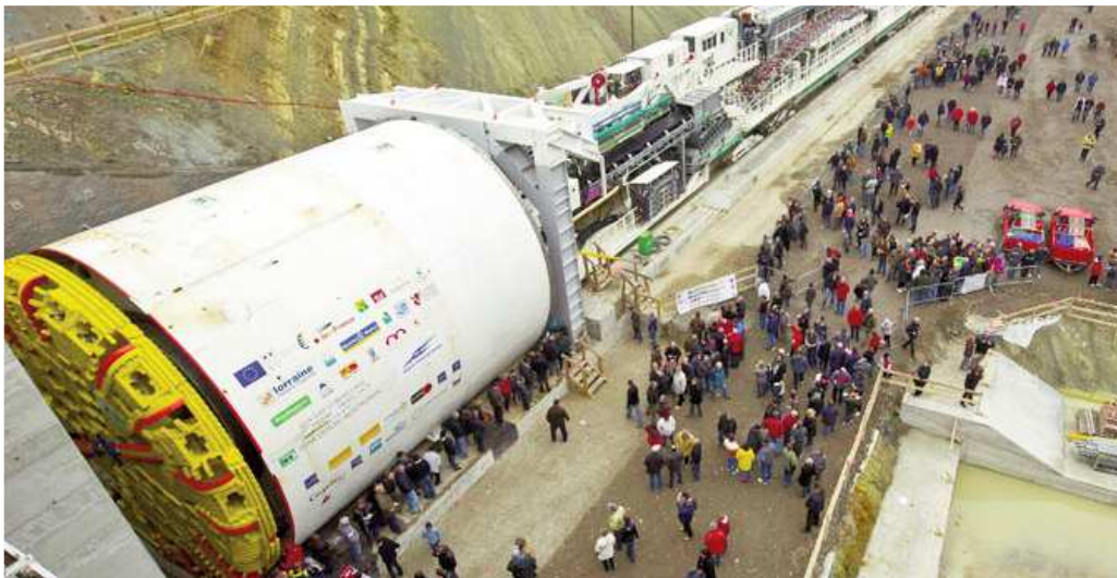
World's Largest TBM: Dual Mode Herrenknecht EPBM at Launch Site
