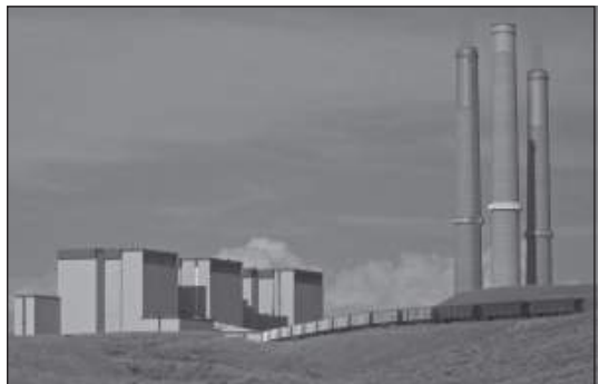
Shutdown for Maintenance, Repairs, Modifications
