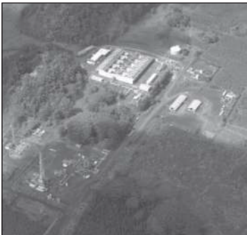
Puna Geothermal Expansion
