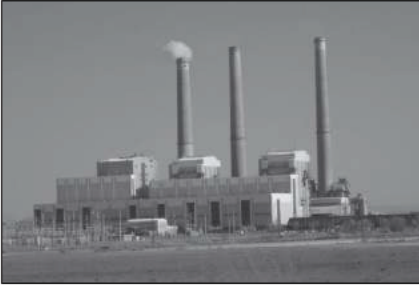
Shutdown to Convert ESP to Baghouse
